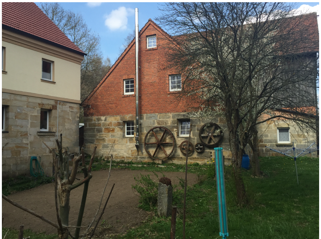
The rear of the Dorfmühle showing the original mill equipment on display – the gears that transferred power from the wooden waterwheel to the grinding stones.
