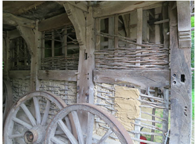
Medieval woven wood walls packed with daub. Daub is a mixture of straw, mud, and manure. Photo Maggie Land Blanck, 2014; Detmold Open Air Museum.
