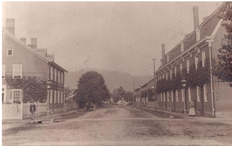
The Great House and Feast Hall, seen on the right in a photo c. 1880. The Harmonists took their meals and celebrated holidays in this building. At the end of the street is the Ohio River.
