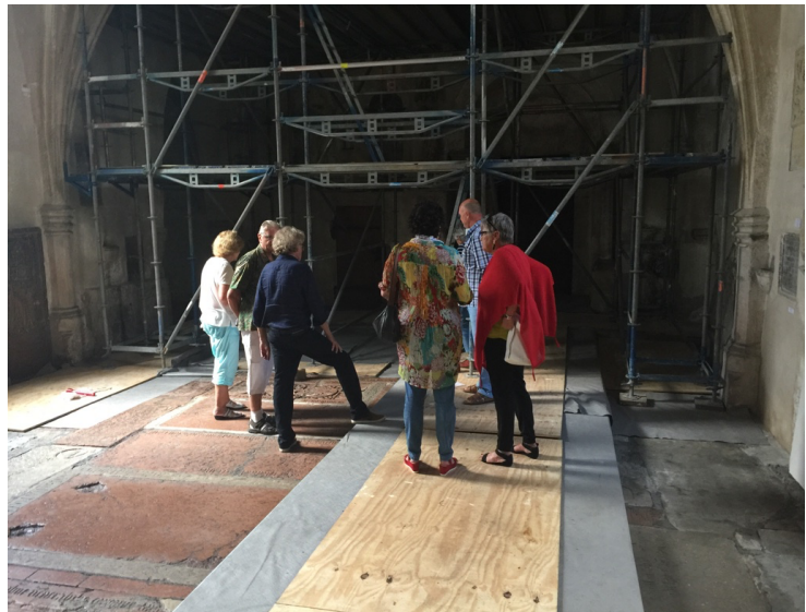
Crypt of St. Peter's Cathedral, Regensburg. In July, 2016, our third cousin Jürgen Dollhopf arranged for a tour of the crypt. The crypt was undergoing restoration at the time. Jürgen, a colleague of the Cathedral architect in charge of the restoration, arranged for special access. In this picture we are standing over the gravestone of Johannes Tolhopf.
